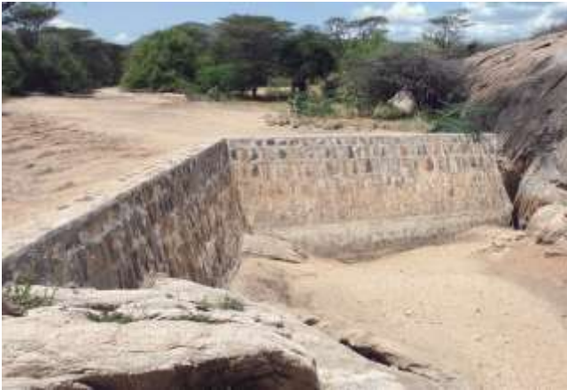
Sand dam in Turkana County
